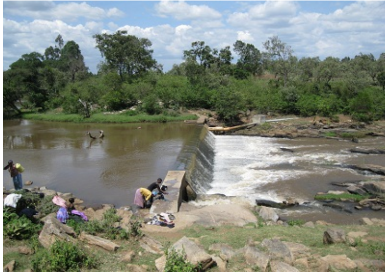
Plate 4.2: A Weir for Chebaraa Irrigation Water Intake at Kaboson Photo taken, 17 th December 2014
